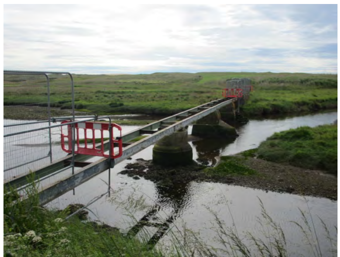
The Spalding Bridge today.
