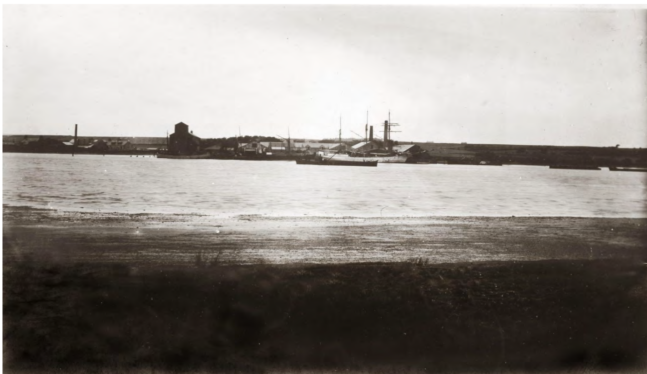
An old photograph of the quay at Newburgh
