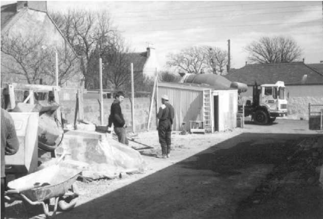
BUILDING THE EXTENSION TO NEWBURGH MATHERS
